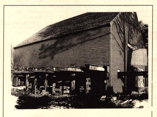
Up in the Air Cribbing and I beams raise the barn to build a new foundation and sill replacement.
